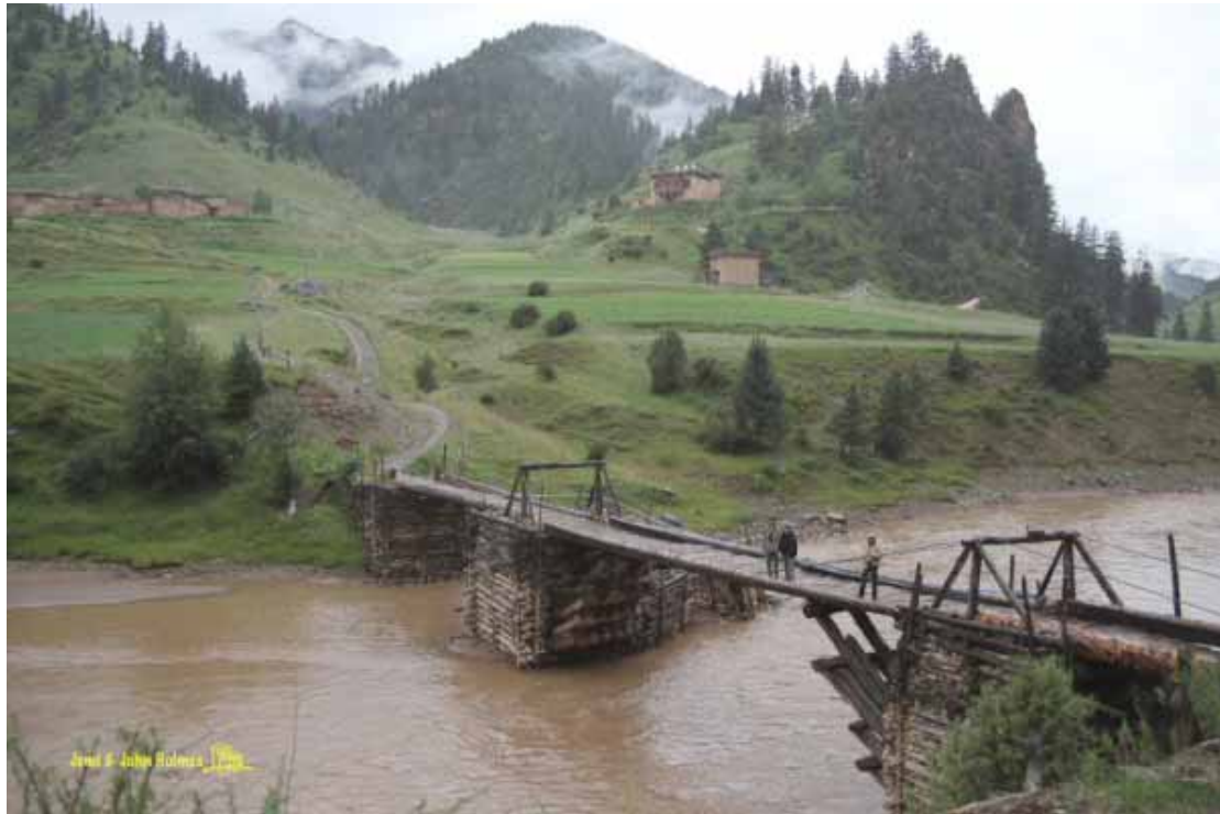
Old-fashioned wooden bridge, Jiangxi Forest Reserve
